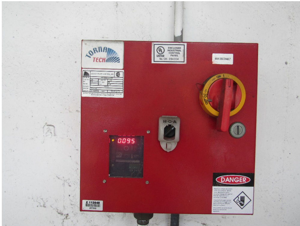
View of the jockey pump controller.
