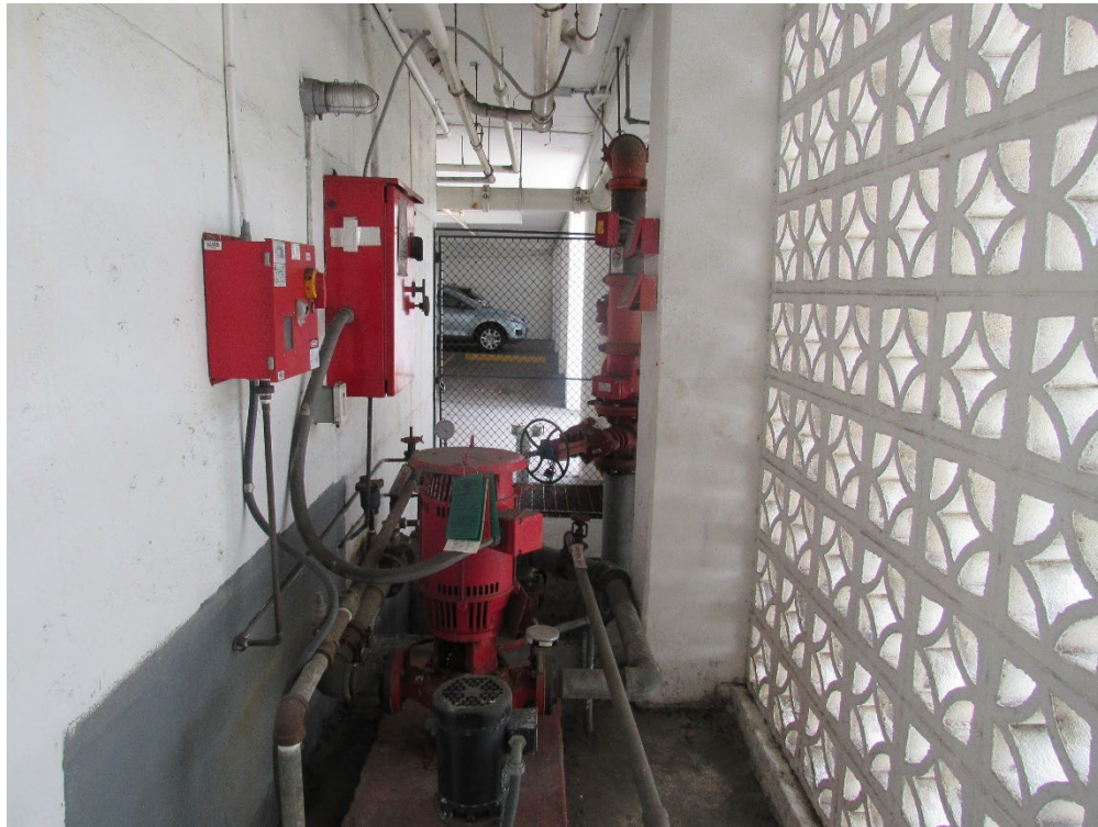
View of fire pump system.
